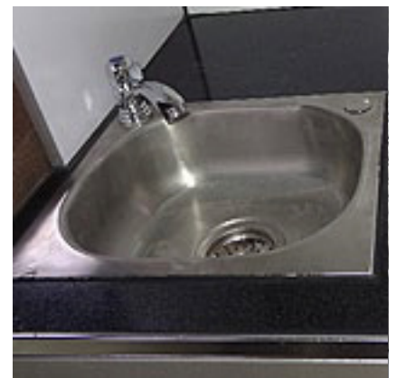
Bench top sink, with 12V pump & stainless water tank underneath
